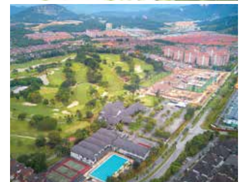
Actual Photo - under construction
